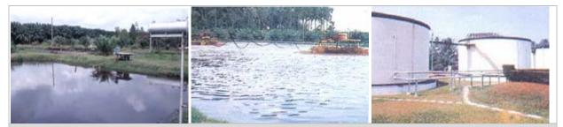
Figure 17 An effluent pond (left), an aerobic pond with surface mechanical aerators, (middle) and anaerobic tank digesters (right).
